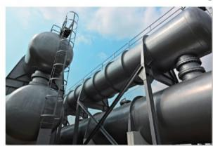
Figure 2 Gas scrubber on an incinerator.
