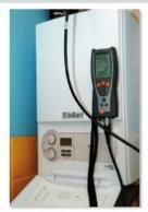
**Figure 4** Gas appliances need to be checked regularly to ensure that they are not leaking carbon monoxide.
